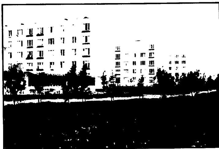
Units completed in 1960 in Moscow.
