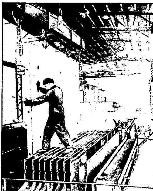
Extraction of a panel from upright molds at a Moscow plant.
