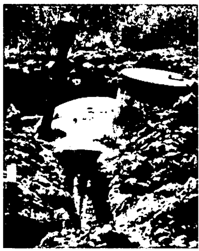
Figure 6. East Germany: Sketch of an Underground "Tank," or "Boiler," Type of Repeater Station in use on "Hardened" High-Capacity Multiconductor and Coaxial Cable Lines and Photographs of Similar Repeater Stations in use in the USSR, June 1960
