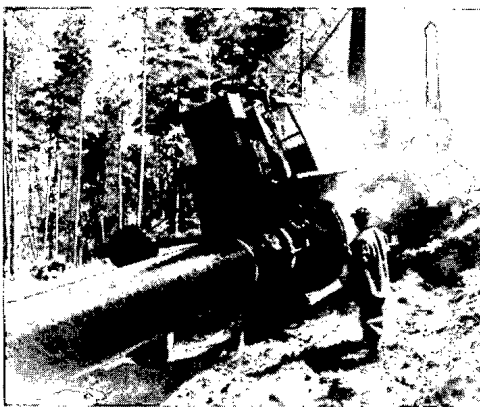
FIGURE 19. USSR: Tuymazy-Irkutsk Oil Pipeline Under Construction.
