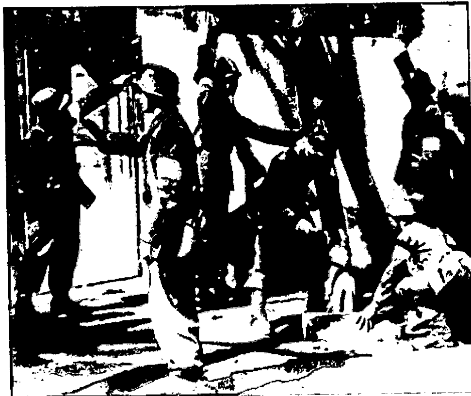
Figure 2. HUNGARY: Civil Defense Students Shoring a House Wall
