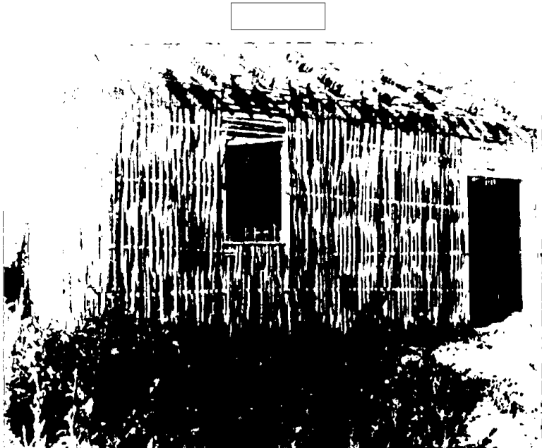
Figure 10. Communist China: Light Bamboo Wall Construction Before Plastering.
