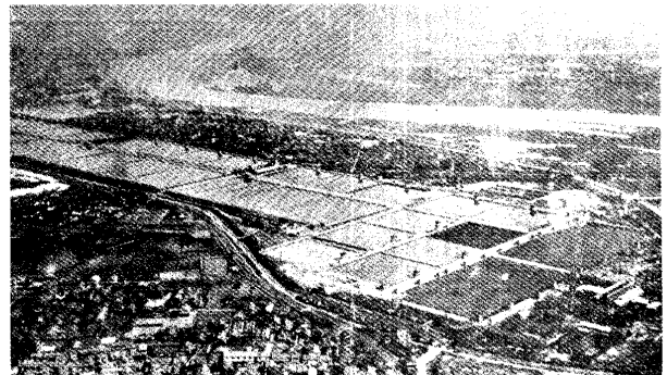
FIGURE IX - 12. Ōsaka Prefecture. Ōsaka, 1936. Kuniijima water purification plant of Ōsaka's system.
