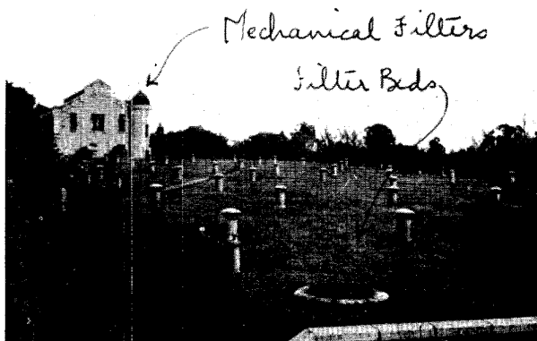
FIGURE IX - 16. Hyōgo Prefecture. Kōbe, date unknown. Okuhirano waterworks of Kōbe's system. Building houses mechanical filters; slow sand filters in foreground under cover. The protruding pipes are ventilators.
