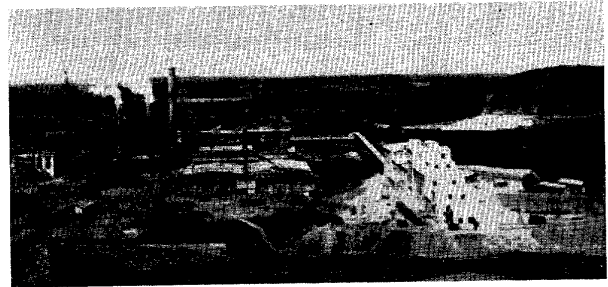
FIGURE IX - 17. P'yongan-namdo, Sungho-ri (Shōko-ri) . The plant of the Chōsen Onoda Semento Seizo K. K. (Chōsen Onoda Cement Manufacturing Company), one of Korea's major producers of cement.
