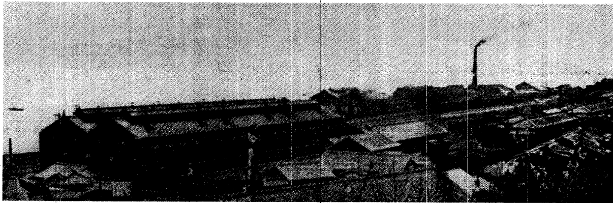
FIGURE VII - 22. Pusan (Fusan) . Pusan Government Railway workshops, before expansion.
