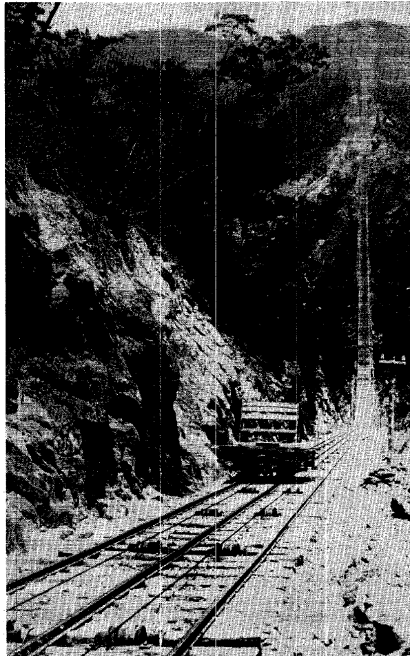
FIGURE VII - 24. Sinhung Railway, Oro-ri to Pujonhoban. North view. Cable railway of the Hungnam (Konan) plant, serving Pujonhoban reservoir. Car of 5-ton capacity. Before 1935.
