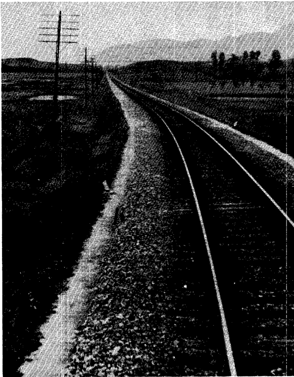
FIGURE VII - 3. Korea Government Railway between Kyongsong (Keijō) and Pusan (Fusan). Roadbed of main Kyongbu line. 1937.
