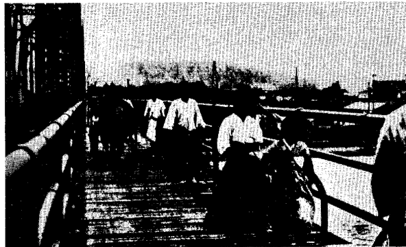
FIGURE VII - 26. Bridge over Yalu river at Sinuiju. Walkway of through-truss railroad bridge. Note vehicle in background. 1935.
