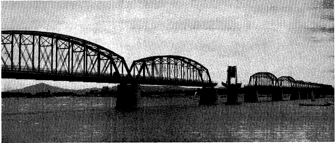
FIGURE VII - 5. Yalu River between Sinuiju, Korea and An-tung, Manchuria. Steel truss swing bridge. Now paralleled by double-track railroad bridge.
