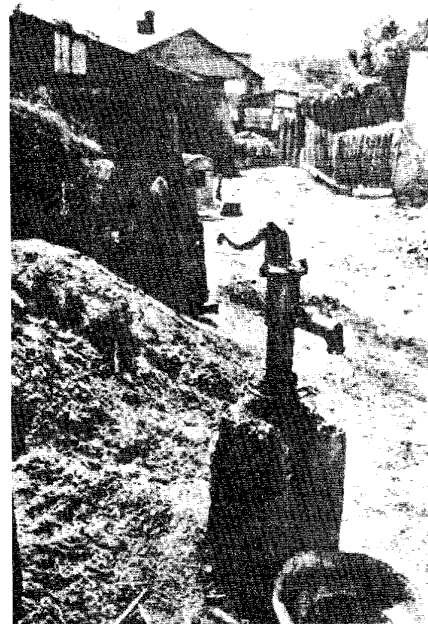
FIGURE VIII-8. Typical village water supply pump. Before 1940.
