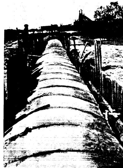
FIGURE VIII-92. Leningrad. Laying of the new sewer at the Krasnyy Oktyabr Stadium. Before 1934.
