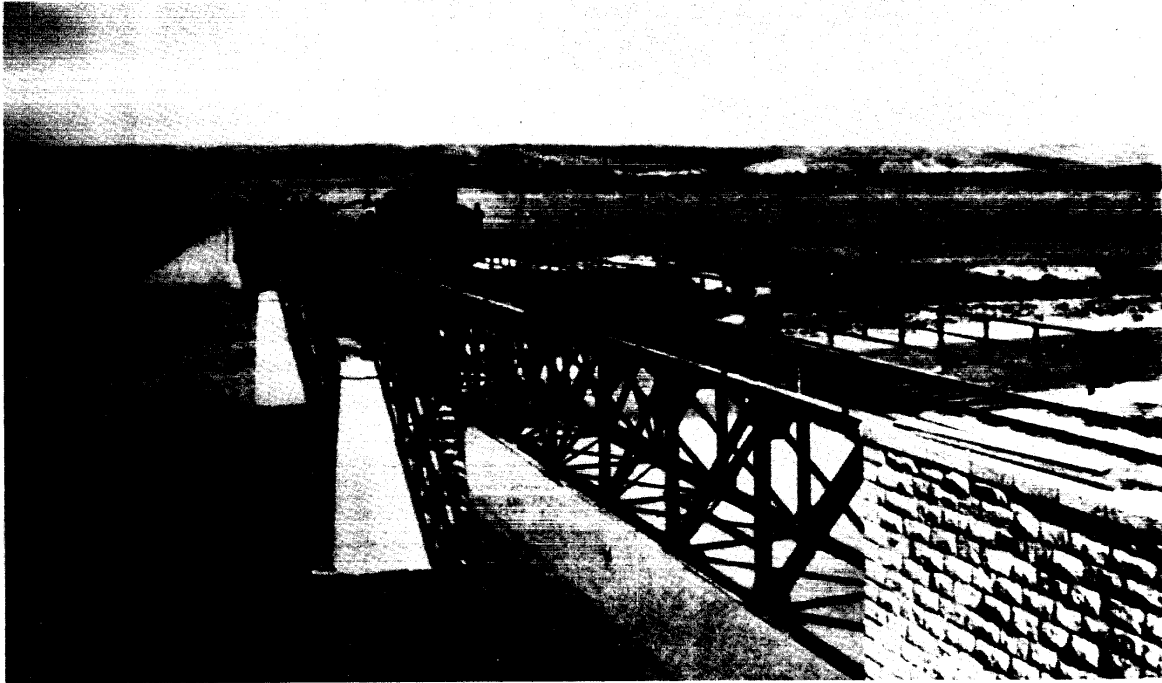
Illustration VII - 9. Yantra Bridge near Bela. Looking westward. 1917. (Bridge 36, line 17.)
