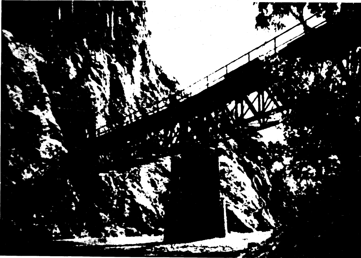
Illustration VII - 3. Cherepich Bridge. Bridge over Iskr River near Mezdra. Tunnel at left. (Bridge 20, Line 2.)
