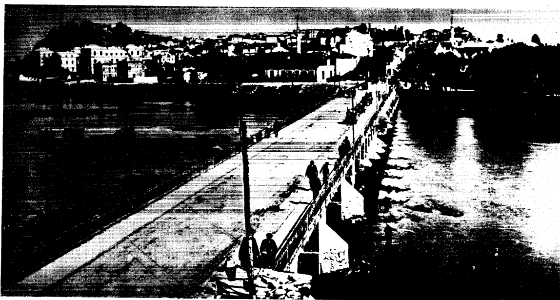
Illustration VII - 30. Bridge over Maritsa River. Road into Plovdiv. Looking south.
