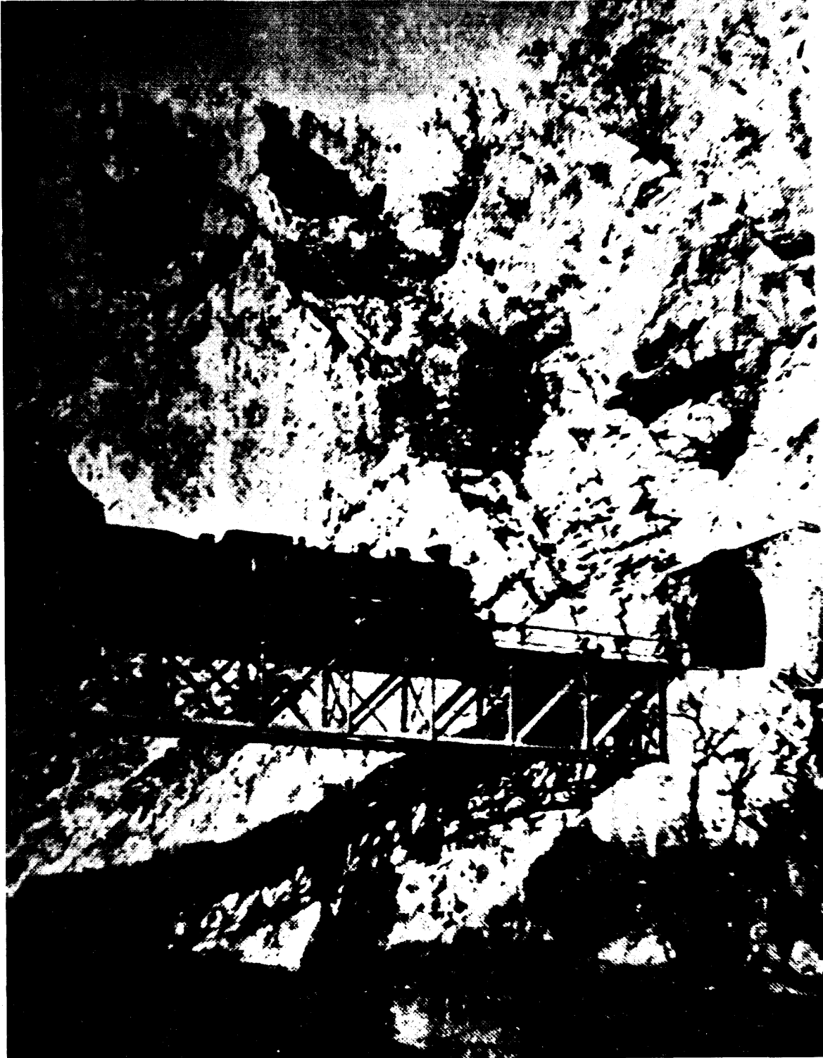
Illustration VII - 2. Cherepich Bridge. Bridge over Iskr River, near Mezdra; railway tunnel at right. (Bridge 20, line 2.)
