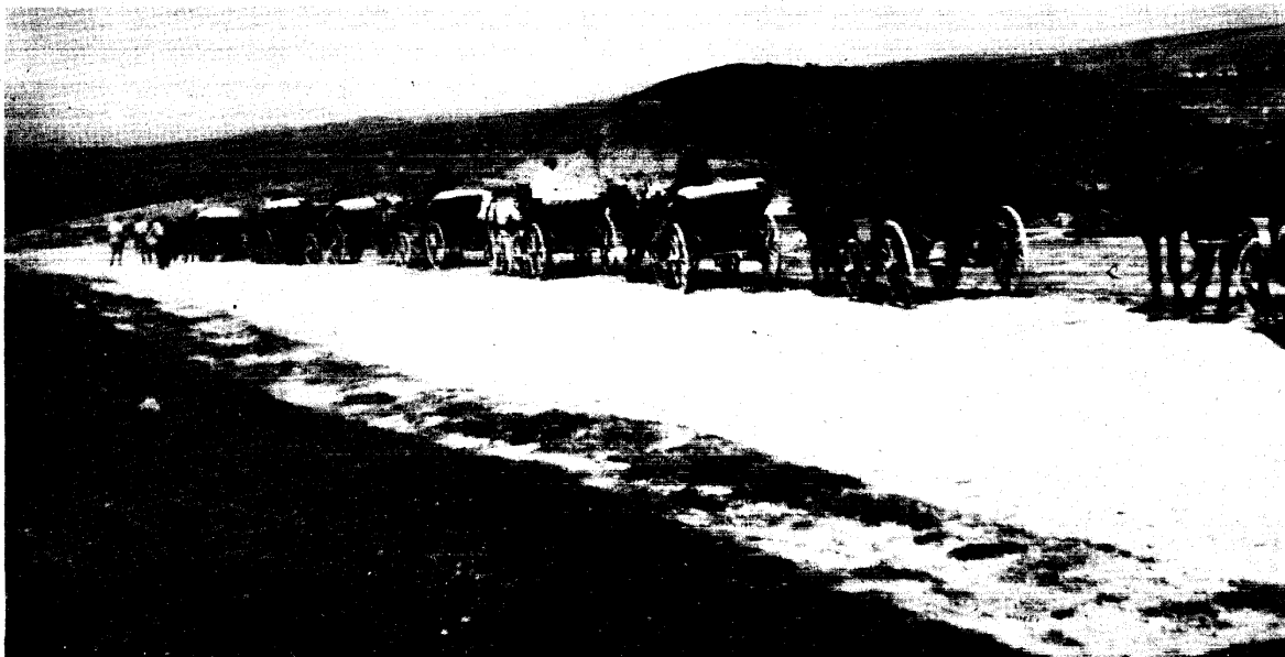
Illustration VII - 23. Minor road near Trnovo. Road leads from railroad station to village in valley.
