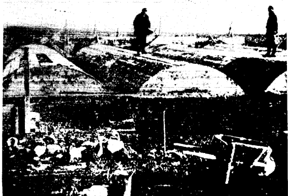
Illustration VI - 18. Burgaz water supply. Construction of the low-level reservoir. November 1925.
