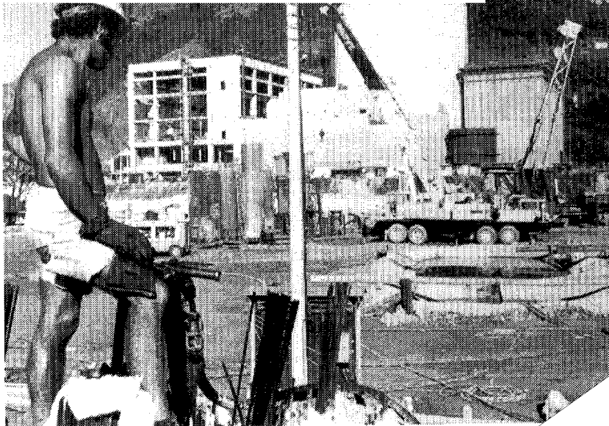
Nuclear plant under construction in central Brazil
