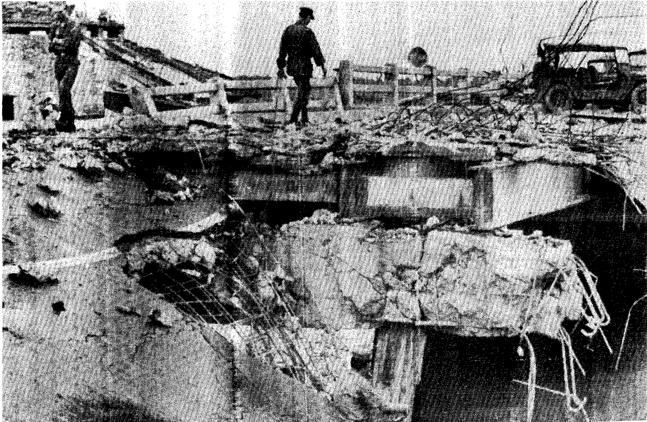
Main bridge on Highway 1 near Saigon
