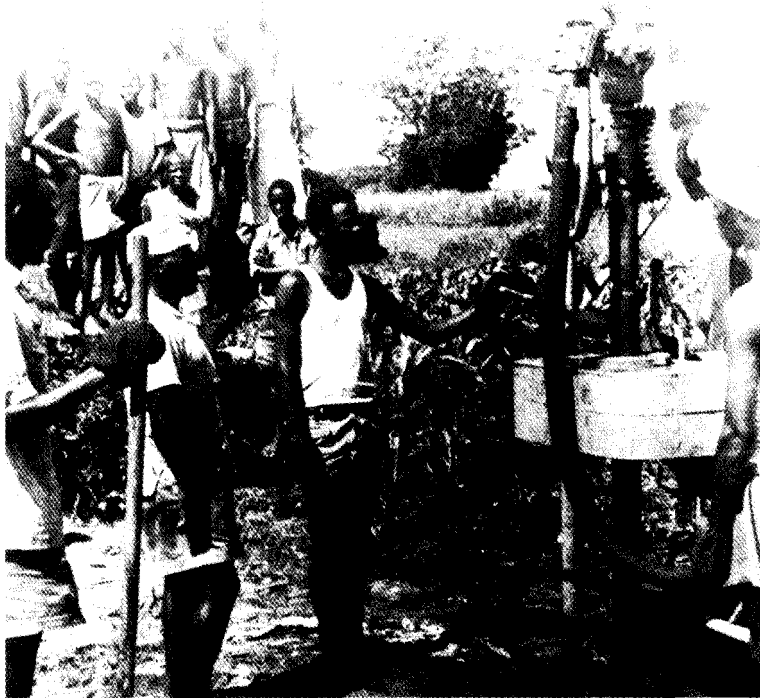
Soviet-assisted Fanole Dam and Irrigation Project in Somalia.
