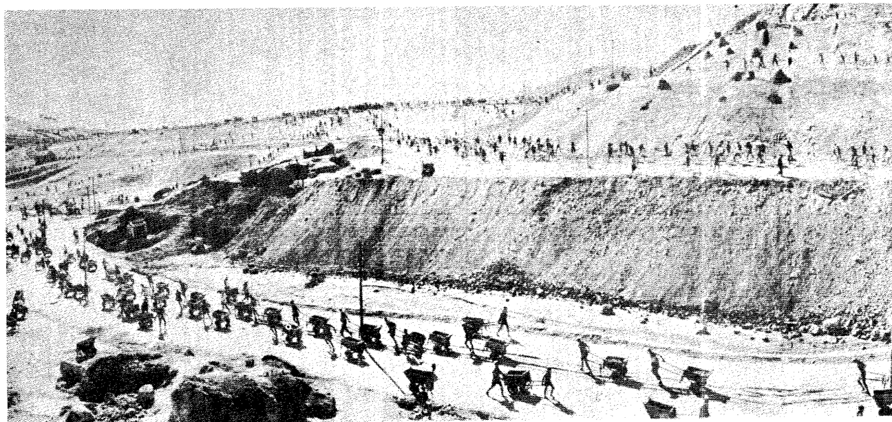
PHOTO OF CHINESE DAM BUILDING PROJECT PUBLISHED IN WARSAW'S SWIAT, 12 OCTOBER 1958
