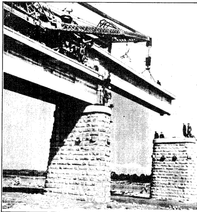
Bridge construction on the Paochi-Chengtou line, using a 65-ton Soviet-type crane built in China.
