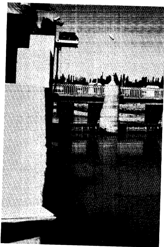
Figure 6. Ferghana Valley. Big Ferghana Canal headworks water level measurement. Note selsyn motor in top left.
