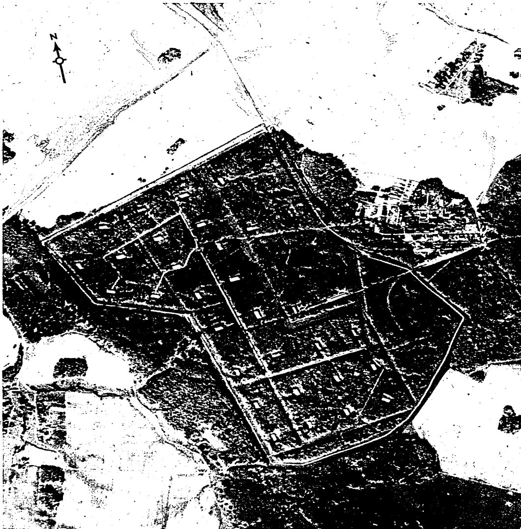
FIGURE 2. KOLOMNA AMMUNITION DEPOT WEST-SOUTHWEST, KOLOMNA, USSR.
