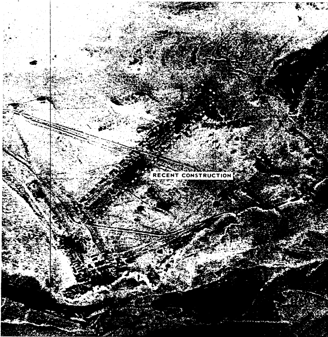
INSTRUMENTATION SITE 13, SARY SHAGAN AMM TEST COMPLEX, USSR.
