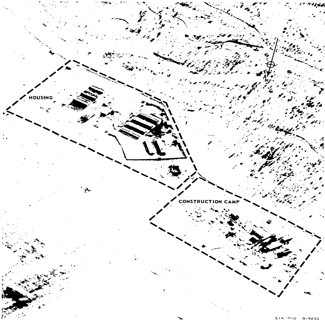
FIGURE 3. SUPPORT AREA "A". The area contains housing facilities, a steam plant under construction, and a construction camp.
