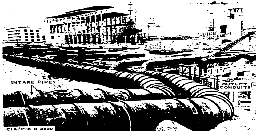
FIGURE 5. PART OF WATER INTAKE AND OUTLET SYSTEM UNDER CONSTRUCTION. The intake pipes are approximately in diameter, and the sections of outlet conduit are approximately . Date of photography August 1959.
