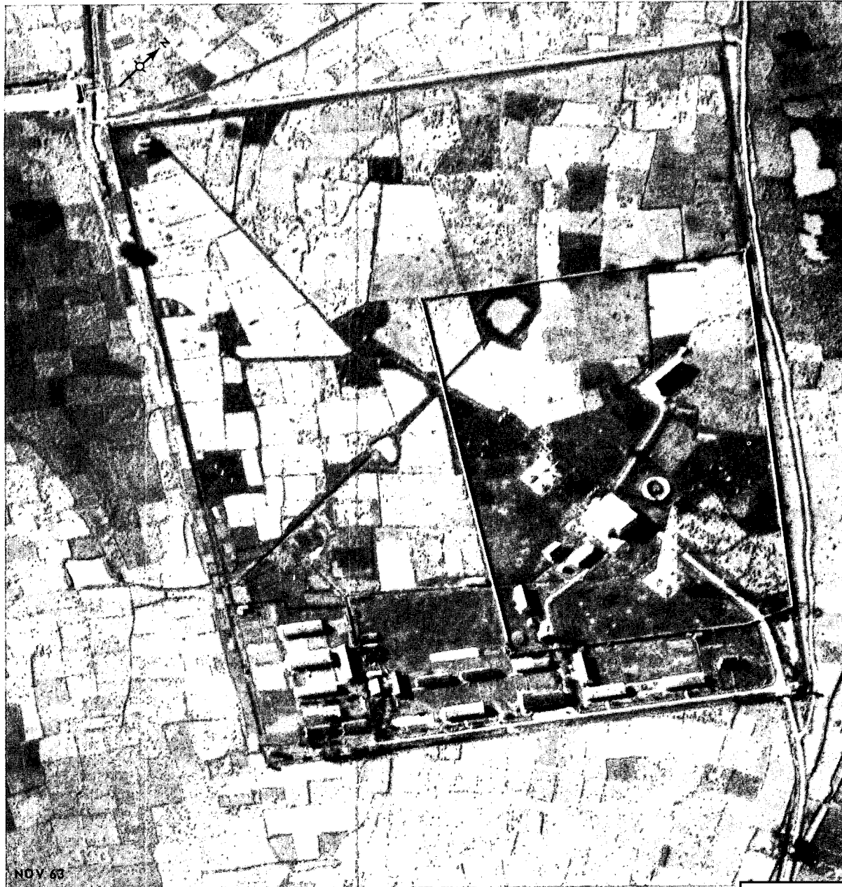
FIGURE 6. HANOI-ME TRI INTERNATIONAL BROADCASTING STATION.
