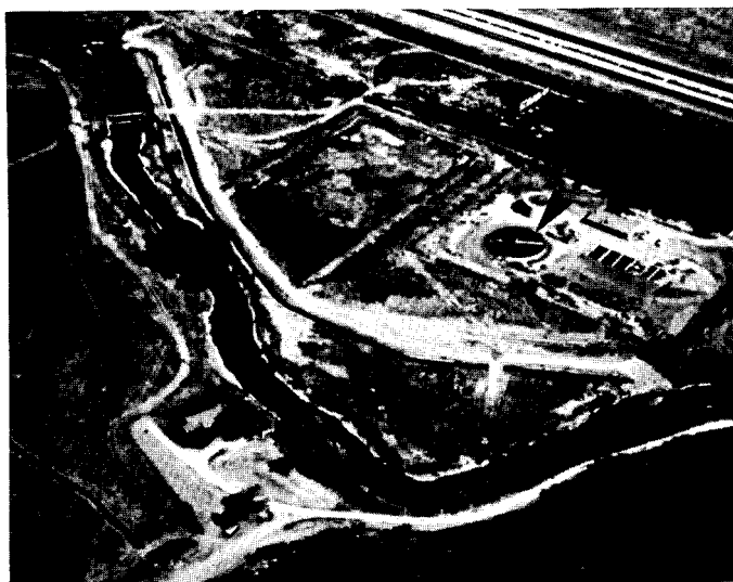
Figure 9.- Beds of trickling filters of overloaded treatment plants, especially those with serious odor problems like this one near Milpitas, California, reflect considerable amounts of infrared energy. The cause of this condition is not known to this investigator - yet. (Note: This condition is quite vivid in imagery obtained using Kodak Ektachrome Infrared Aero Film, Type 8443, from which this illustration was copied.)
