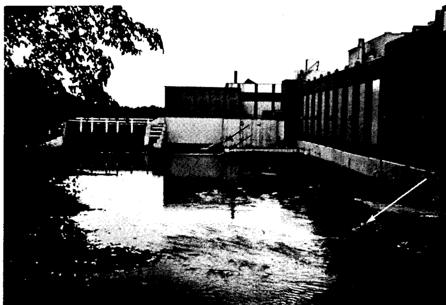
Figure 12.- Spent sulphite wastes from the Blandin Paper Company plant at Grand Rapids, Minnesota being discharged into the Upper Mississippi River. Sickly green sulphite wastes and scummy paper fiber discolored the entire river for several miles downstream when this picture was taken in the summer of 1961.
