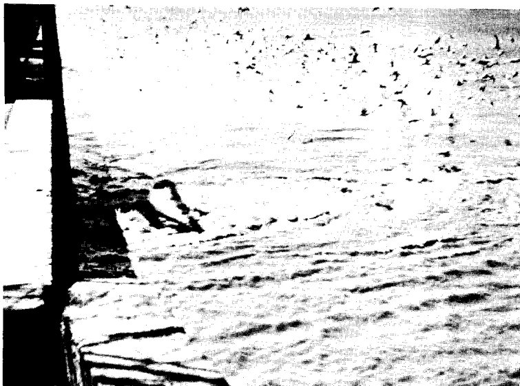
Figure 5.- Raw sewage being discharged into the Potomac River just upstream from the Lincoln Memorial in Washington, D.C. During 1963, raw sewage was discharged from this and 70 other outfalls along the Potomac and Anacostia Rivers an average of 5 days each month, as cited in a report issued by the Senate Public Works Committee.
