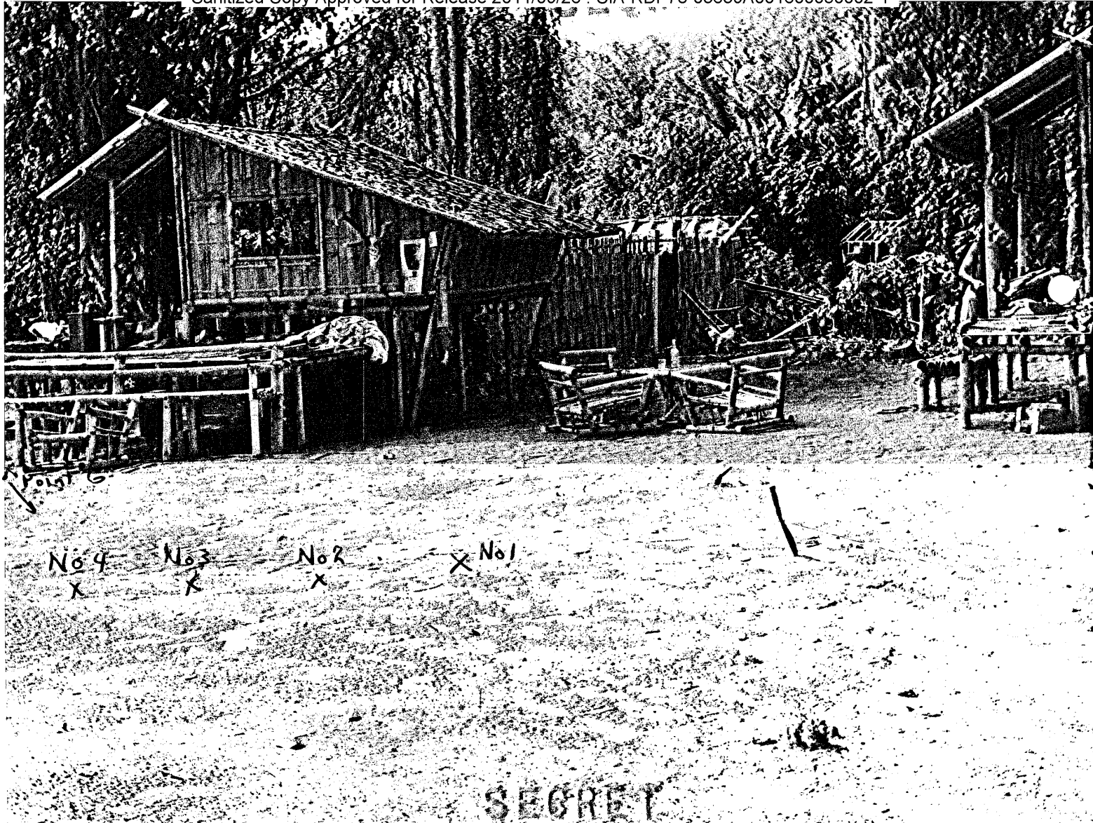
Photo "K" Looking from point F, Photo I toward guest house. Where caches are located.
