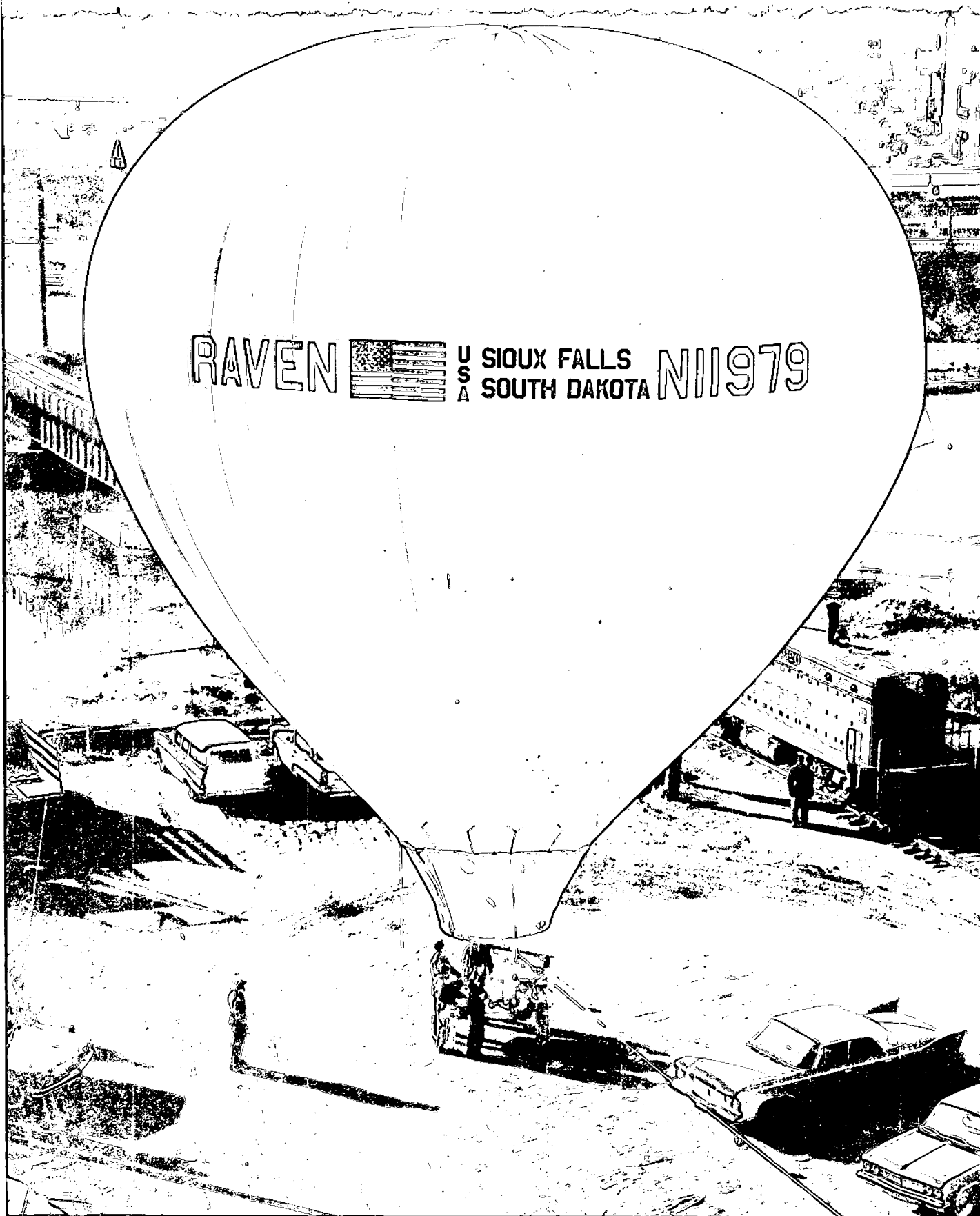
Figure 5 - CA-50 Balloon, made from Nylon Coated with Acrylic
