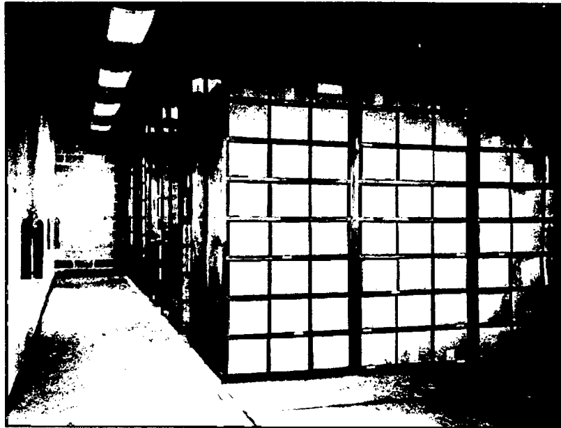
Figure 3. Underground Space Occupied by the Vital Records Depository, Exterior and Interior Views
