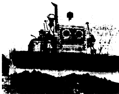
Tractor-dozing moving earth during construction of culverts for flapgates.
