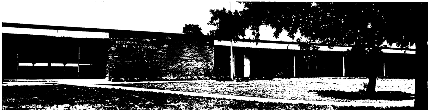
Bendwood Elementary School, Houston, Texas Architect: H. C. Will and Koetter and Tharp, AIA Mechanical Contractor: Glenn H. Engbrock, Inc. Acoustical Contractor: Straus Frank Company
