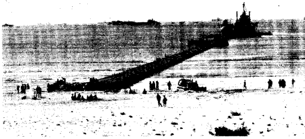
LST married to 1620 ft. Pontoon Causeway Pier (longest on record) at Huelva, Spain.
