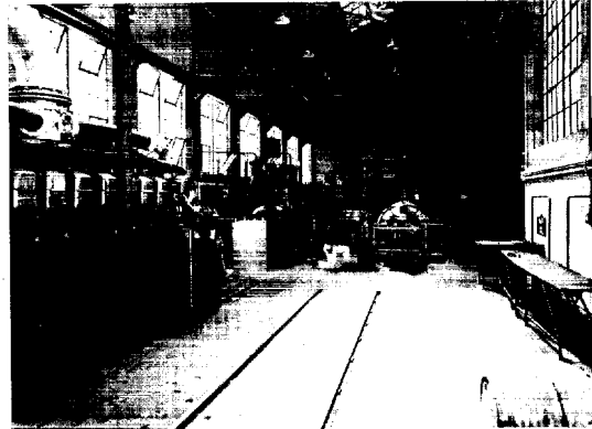
PART OF THE THERMAL POWER STATION AT NOVA LISBOA
