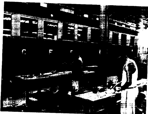
THE CARPENTER SHOP AT NOVA LISBOA
