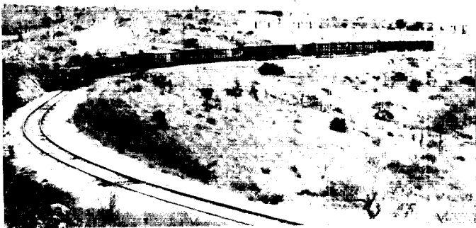
"MOUNTAIN" GARRATT LOCOMOTIVE PULLING A TRAIN ONTO A SIDING AT PORTELA AFTER CLIMBING NEARLY 300 METERS IN 12 KM. NOTE THE TYPICAL SHORT LENGTH OF THE TRAIN.
