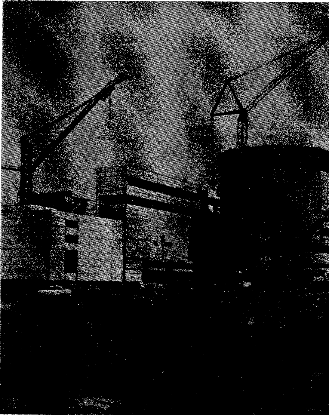
Fig. 1. Fiftieth-Anniversary-of-the-USSR Novovoronezh nuclear power station: the construction site for the fifth block with 1000-MW vessel-type reactor. Construction should be finished in 1978. In the future, blocks of this type will form the basis for the increase in power of nuclear power stations with vessel-type reactors.
