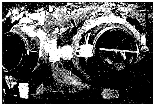
Fig. 3. Reactor-vessel nozzle area with stamped-out nozzles DU-850 in a VVER-1000.
