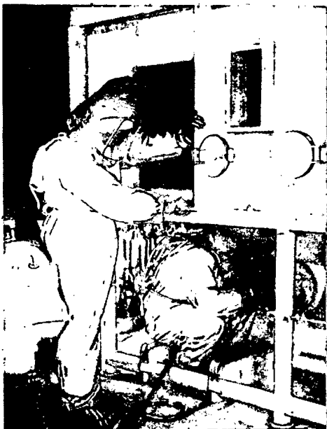
Fig. 1. Maintenance work in progress on heavy cells, with personnel dressed in pneumatic suits type LG-2.
