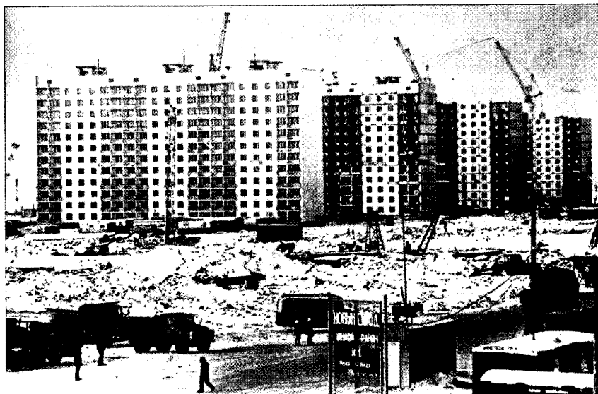
Worker housing under construction at the Kama River industrial complex near Naberezhnyye Chelny
