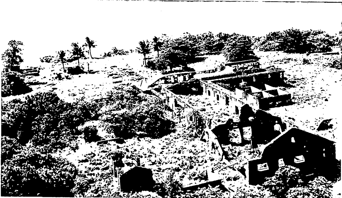
Ruins of Japanese-built facilities on the east end of Itu Aba.
