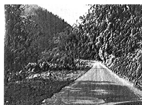
Figure 5 Interlevel bituminous surface on LOC Route IX between Nepal, India and Kanak, Nepal, 1963 (U)
