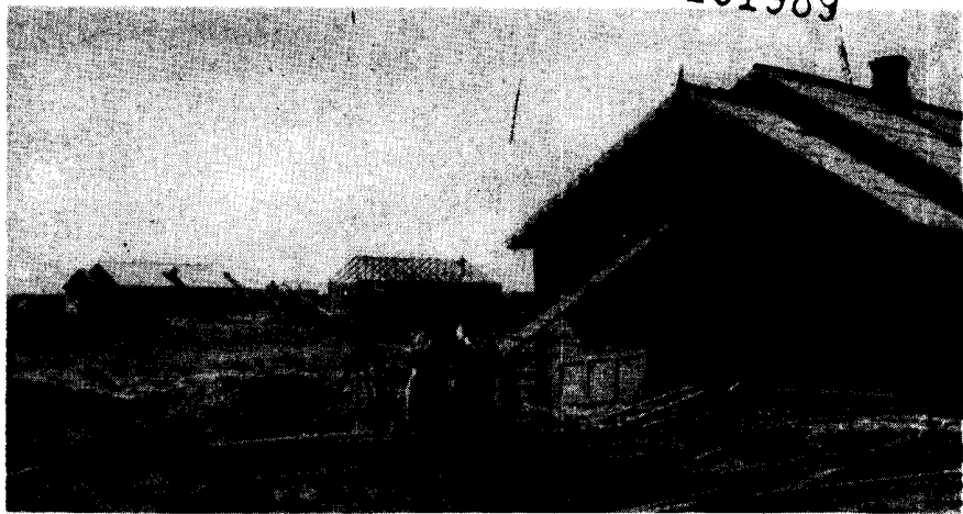
HOUSEBUILDING AT TAKHIA TASH. Construction workers have moved into the area to put up houses for the members of the project's permanent staff.
