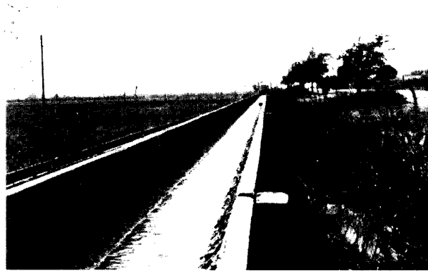
Open irrigation ditches are used throughout the Bled to move water. Much scarce water is lost through evaporation.
