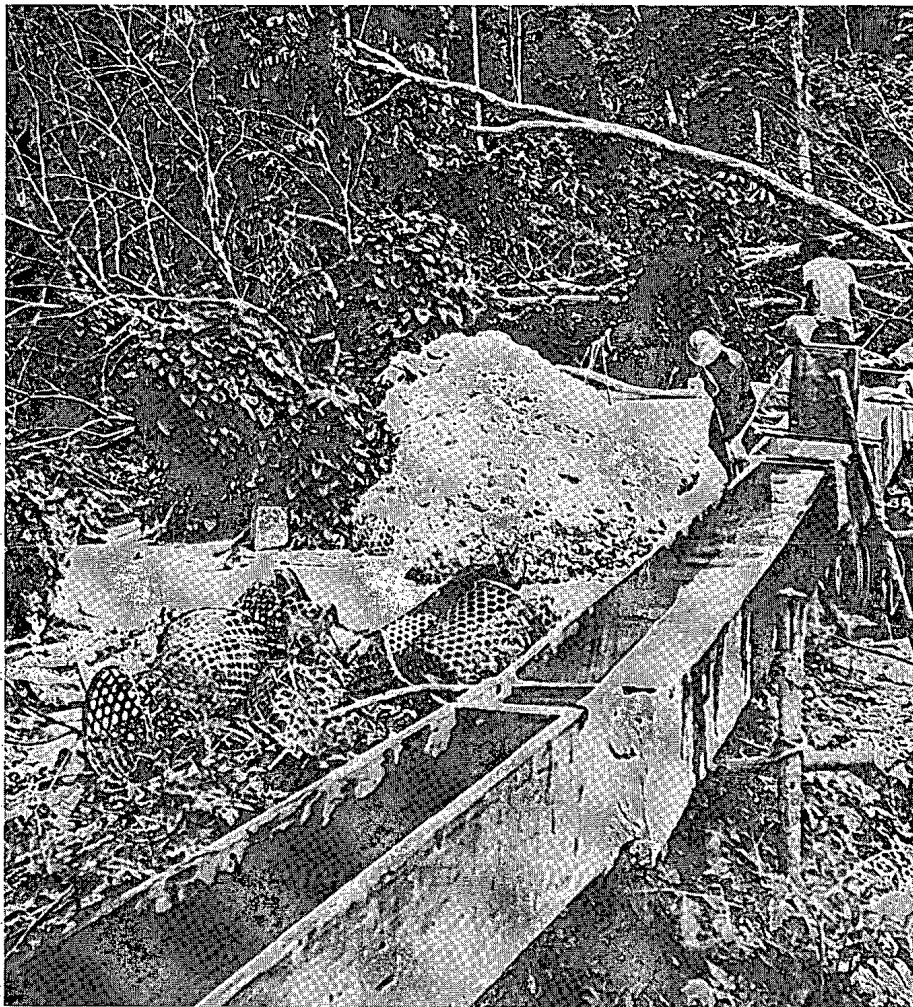
FIGURE 7. Primitive sluicing operation for washing gold-bearing alluvial sands.
