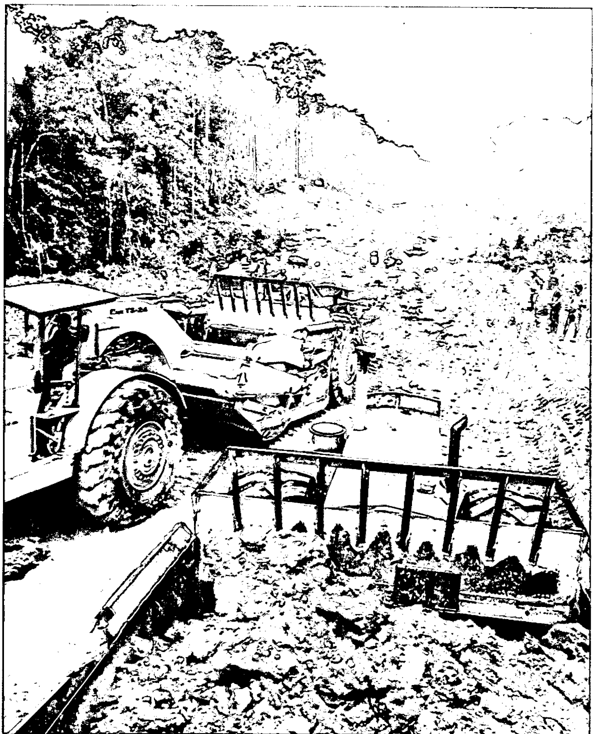
FIGURE 13. Heavy construction equipment must be used to capacity during the less rainy period when the heavy red clay soils are more manageable.
