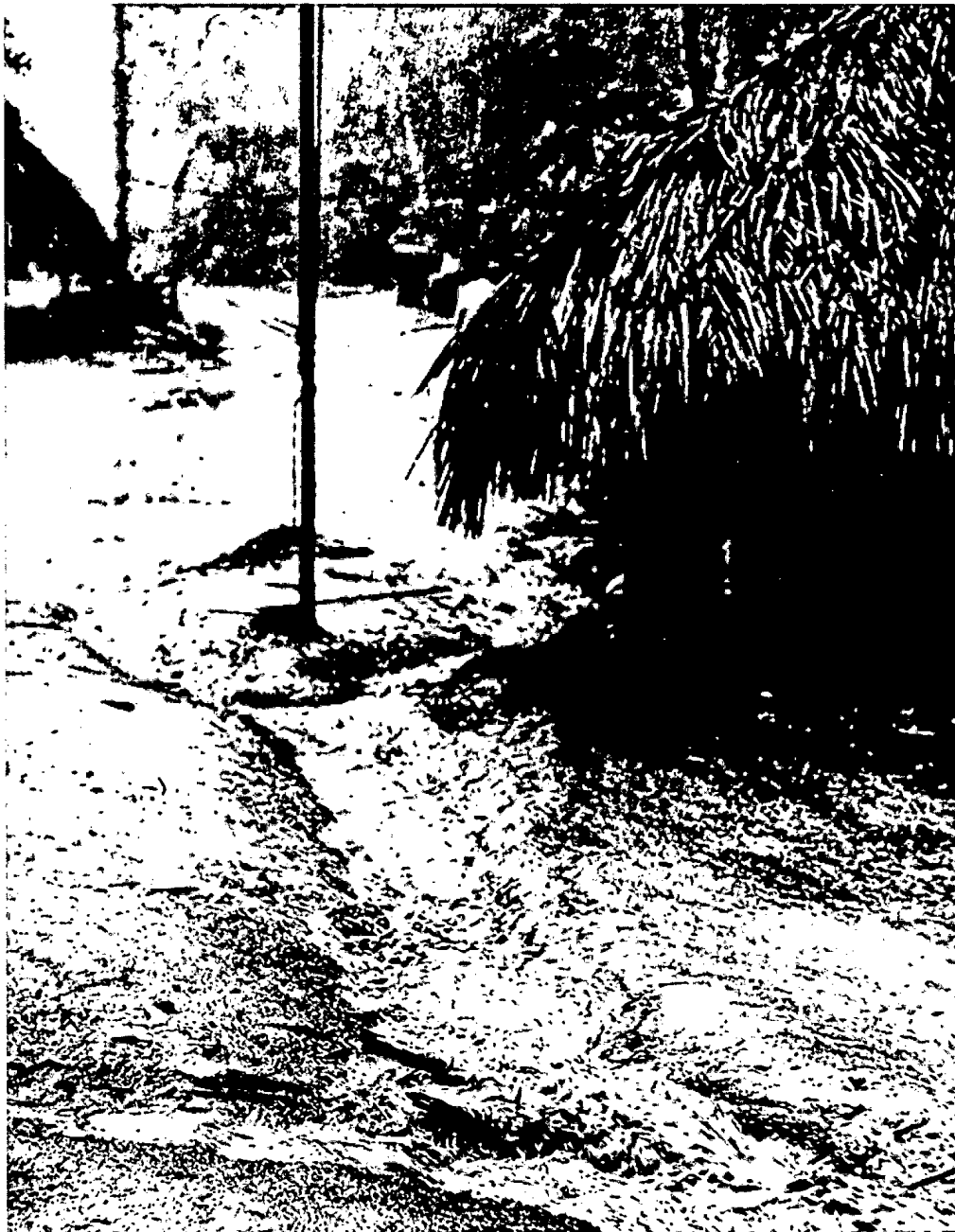
FIGURE 17. Bare ground quickly erodes under the powerful onslaught of tropical downpours.
