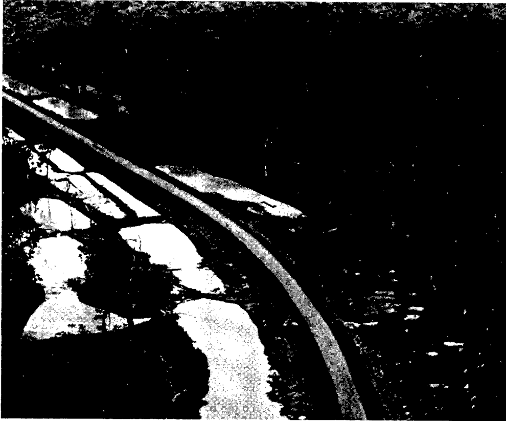
FIGURE 15. Surface drainage has been a particularly difficult engineering problem in constructing the Manaus-Porto Velho Highway.
