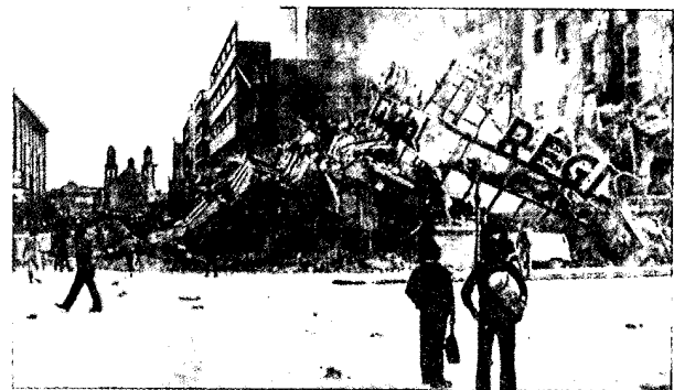
Figure 5. The Hotel Regis was one of several hotels destroyed in the Mexican earthquake. [ ]
