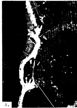
Photo A illustrates a drive-through revetment at VK359032, that is being hardened for use as a possible storage area. This operation is nearing completion, with the roofing nearly intact.
