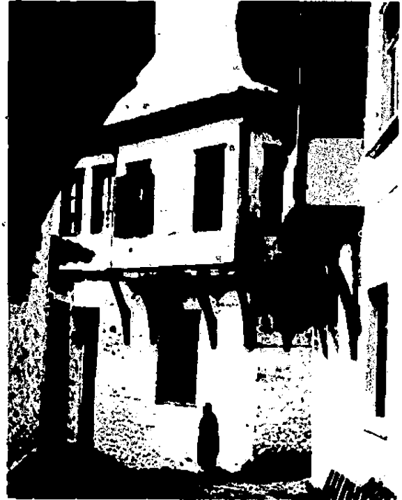
Old houses in Thrace and other parts of northern Greece frequently exhibit Turkish influences, such as overhanging solar
