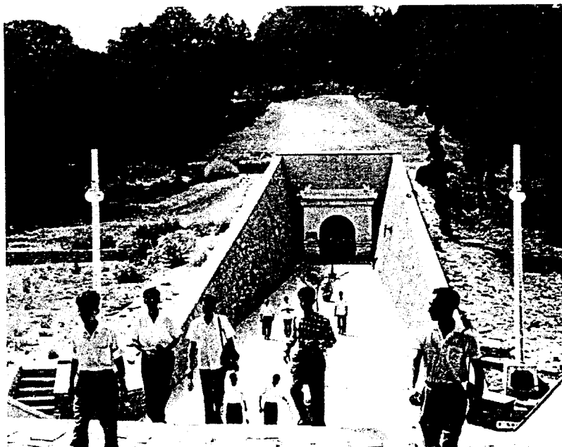
Figure 50. One of the Ming Tombs. This is the entrance to the underground vault of Ting Ling -- the only tomb open to the public.
